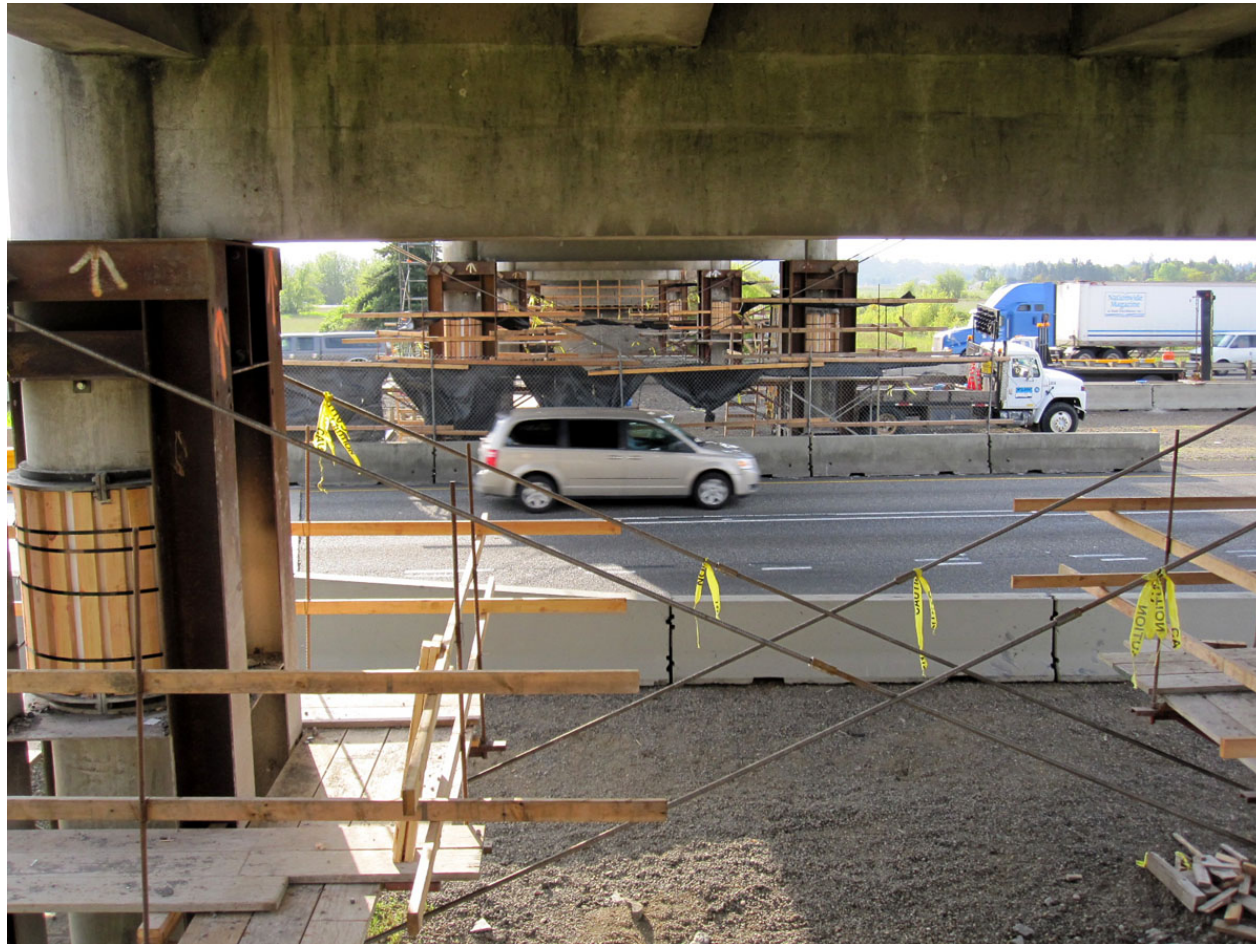
Preparing new column splices
